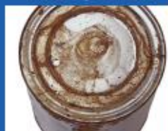
Excessive and pitted rust
