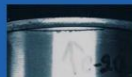
Knocked down flange
